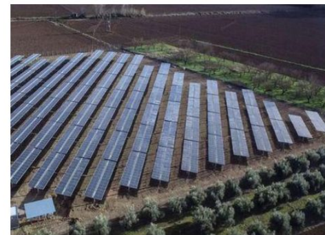
ENIA ENERGY COMMUNITY - KOZANI
